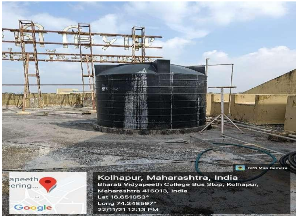
Main building cement water tank No.3
