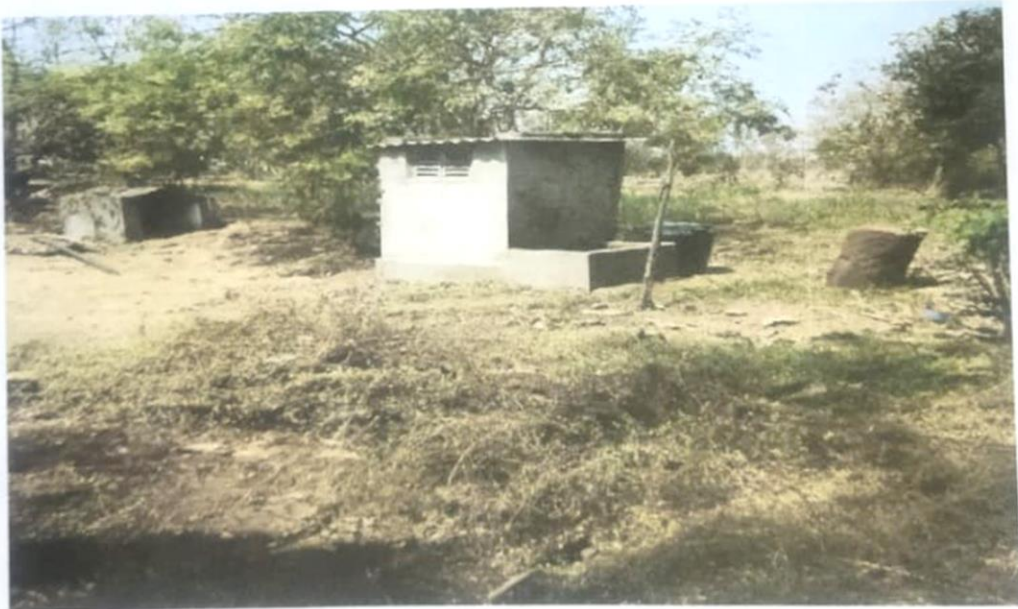
Photos-Biogas Plant at Kandalgaon Kolhapur
