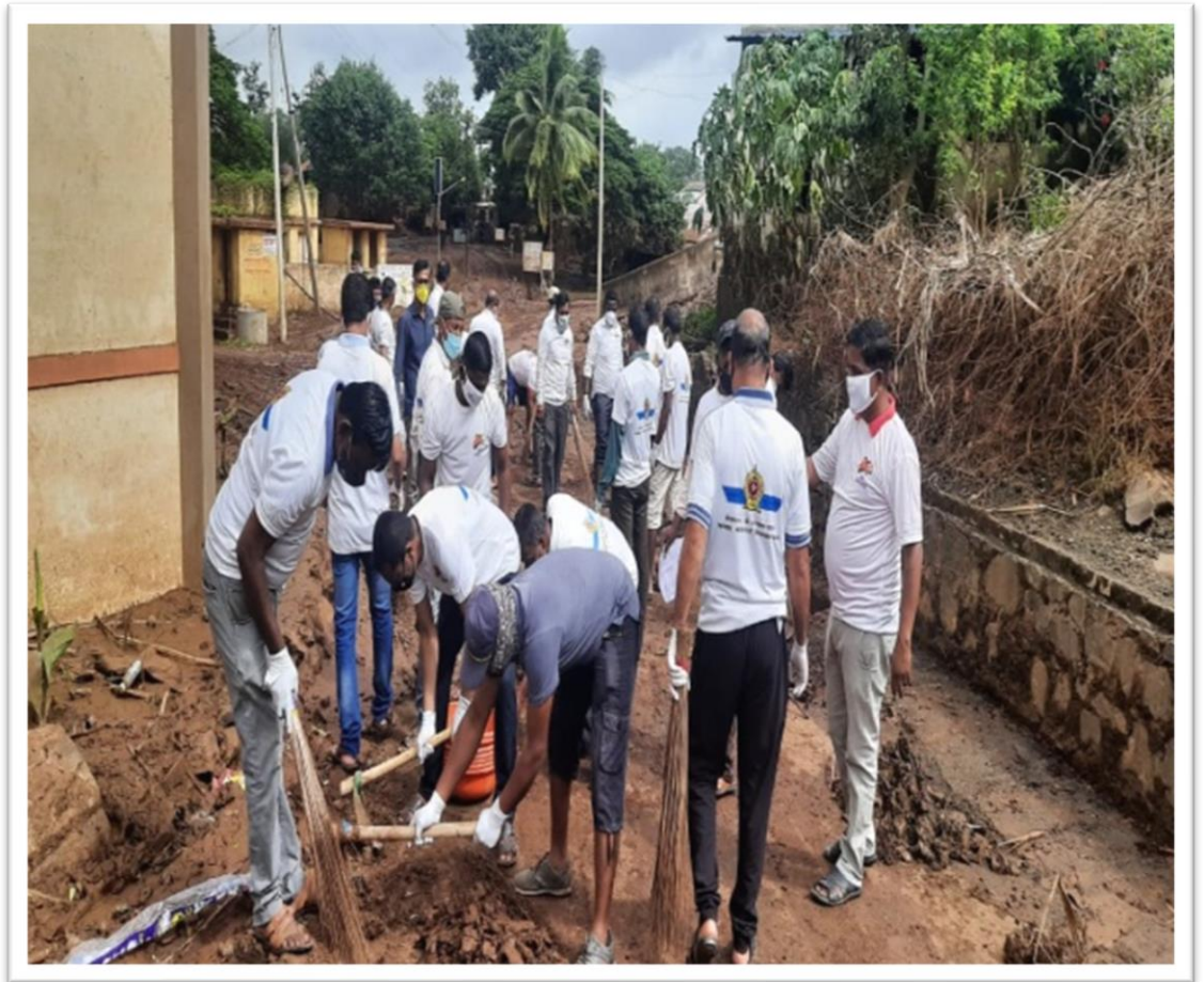
Cleaning of flood affected area in Ankalkhop
