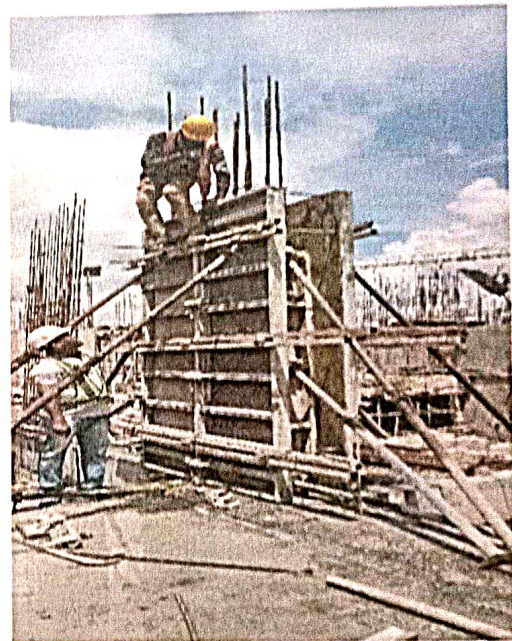
COLUMN SHUTTERING
