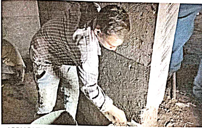
APPLICATION OF WATER PROOFING LIQUID
