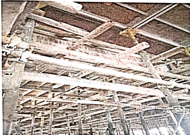
SHUTTERING TO SLAB WITH ADJUSTABLE PROP SUPPORTS
