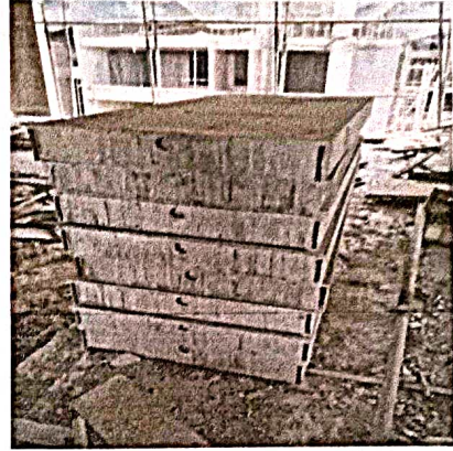
STEEL PANELS FOR SHUTTERING
