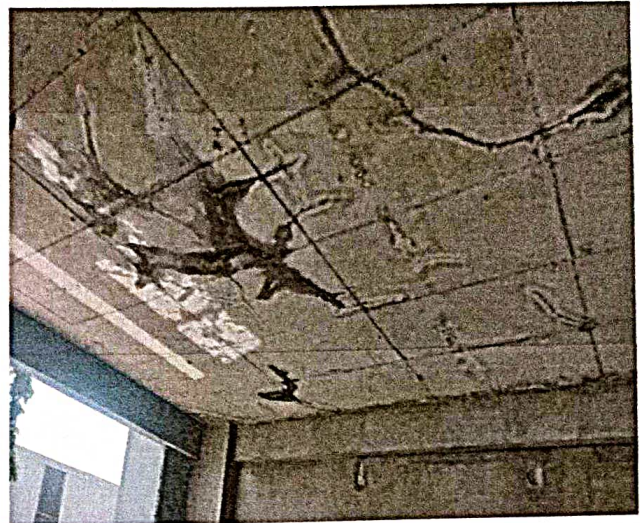
SEEPAGE AND CRACKS IN SLAB
