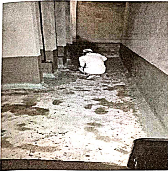
APPLICATION OF WATER PROOFING LIQUID
